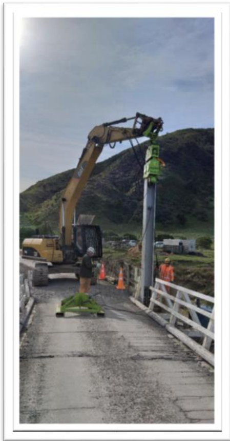
Pile driving Tora farm Settlement bridge.
